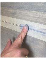
If desired, a deeper grout joint can be achieved by removing material just under the grout joint area with a grinder or scraping tool. Modified grout and caulking grout can also be used.
