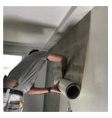
Tips: We recommend to use a roller when pressing to remove air pockets. Repeat process until walls are covered
