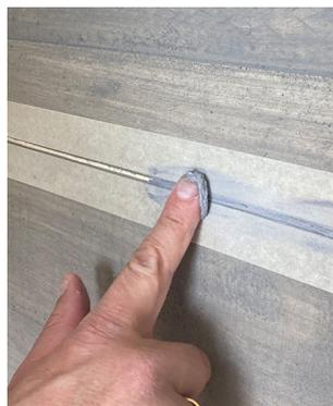
Tests show the use of water based epoxy and acrylic premixed grout work well to fill between the sheets. These grouts are available in several colours to match the existing decor.
